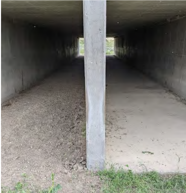
Figure 10 - Existing box culvert
