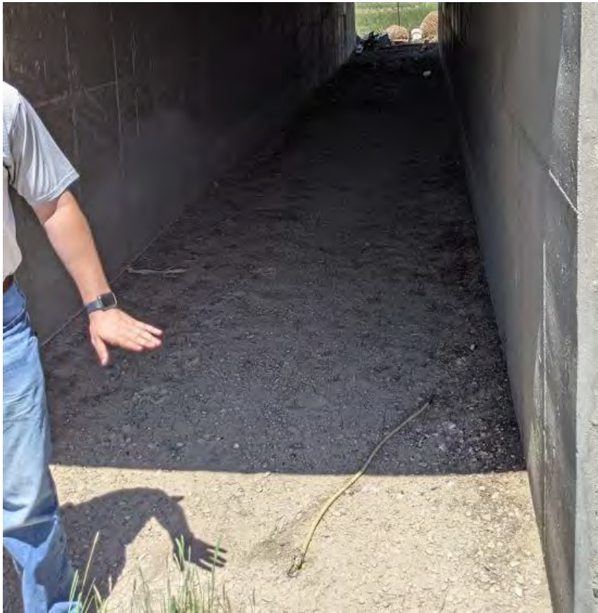
Figure 8- Alignment 1 Existing Culvert
