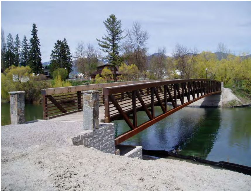
Figure 12- Example Overhead Pedestrian Bridge
